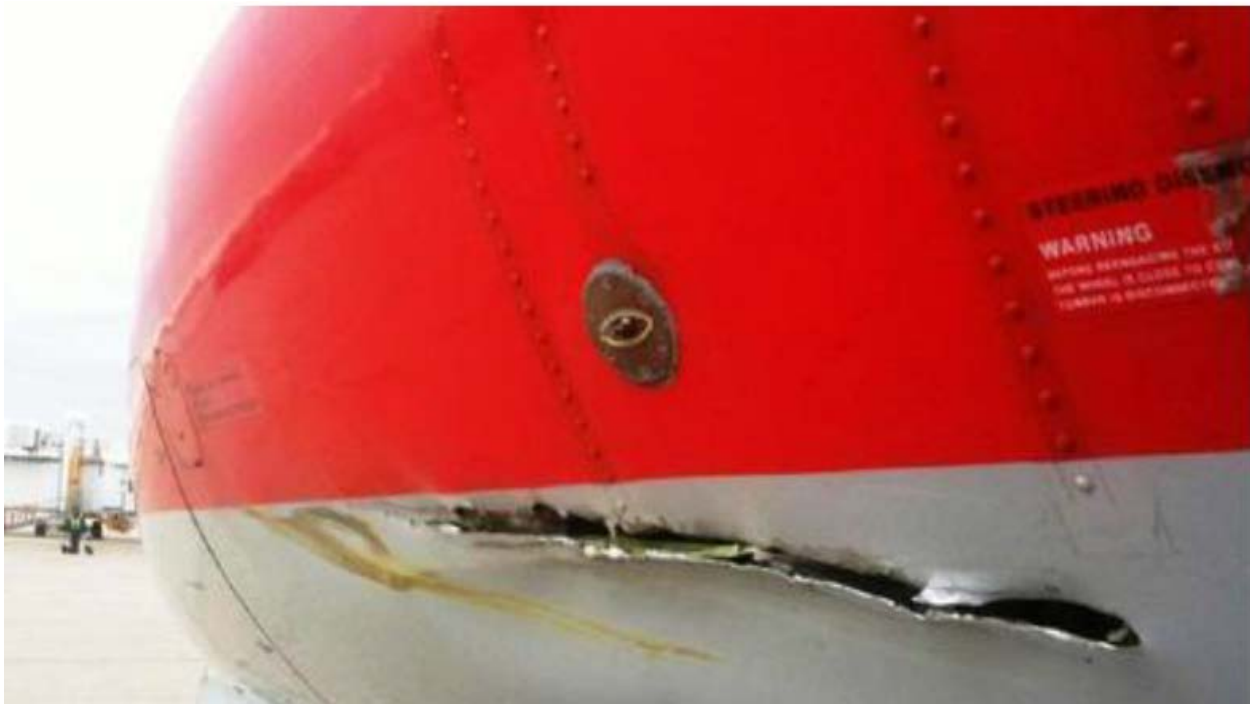
Figure 1: Hole in the fuselage where the PBB struck the aircraft
