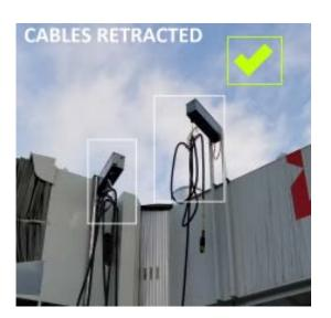
Please ensure GPU cables are fully retrated prior to PBB operation.
